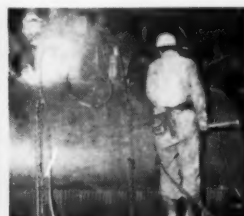
(2) Installation of one-half of steel split sleeve being welded and bolted over old drum core.
